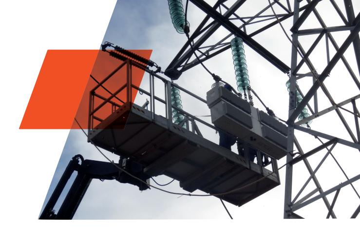
As mentioned above, the circuit on this pilot generally had a low current. This reduced the opportunity for the SmartValve units to deliver operational benefits. This is because the test units were configured to switch on at a minimum current that was often above the typical norms for the test circuit.
