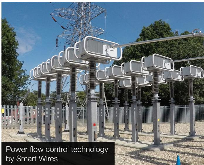
Power flow control technology by Smart Wires
