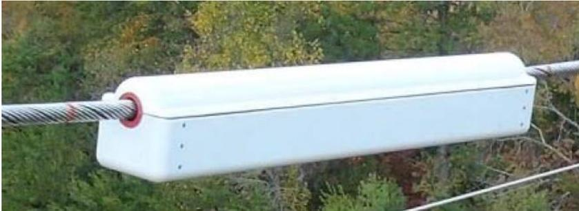
Figure 3-1 DSR on a Transmission Line
