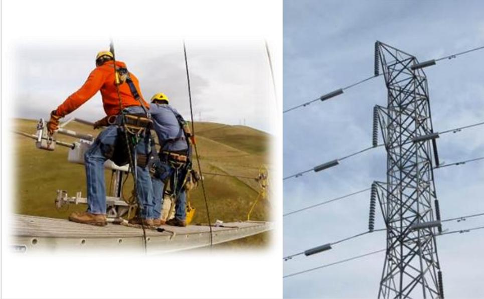
Figure 4-1 Tower on Las Positas-Newark 230 kV line with 6 units installed and Crew Installing Unit
